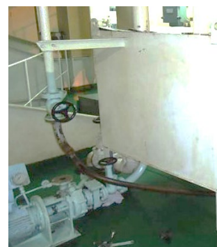
Use of flexible hose to bypass OWS
