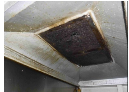
Build-up of grease creating a potential fire hazard
