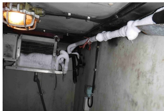
Excessive ice accumulation to pipework and evaporator
